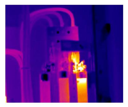
Fig.15 Inspection of connectors
