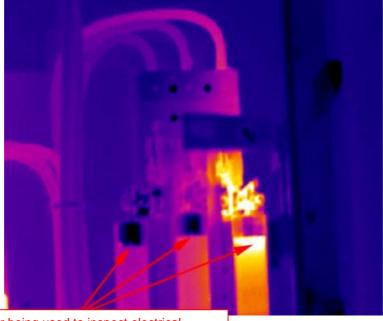
Thermal Imager being used to inspect electrical equipment. With equal load and emissivities the temperature of the three measurement points should be the same.
